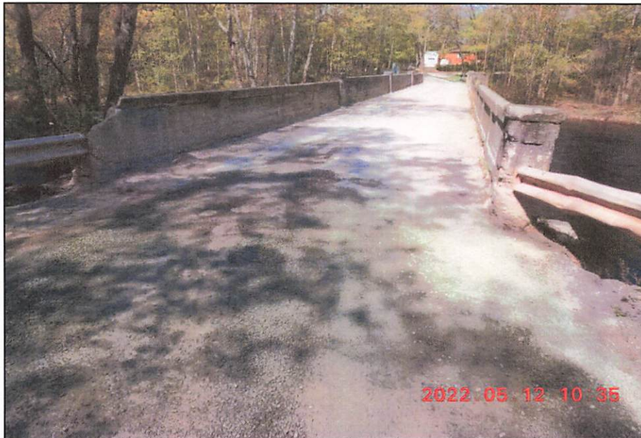
Photo 1: East Approach and Deck Top Looking West
