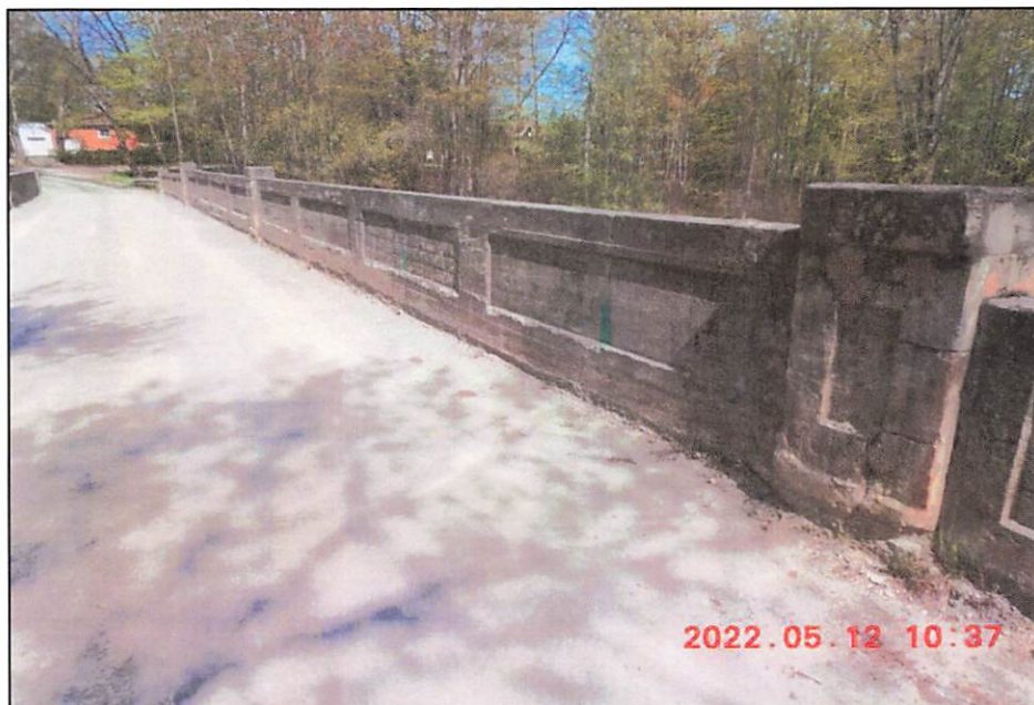
Photo 2: North Interior Barrier Wall Looking West
